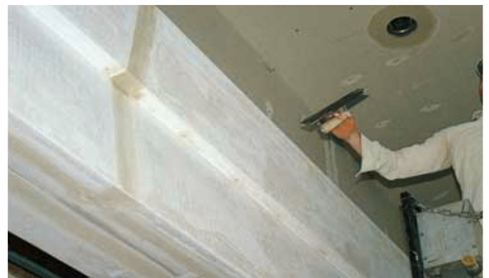
FORMGLAS AND GYPSUM BOARD CEILINGS ARE TAPED AT THE SAME TIME.
